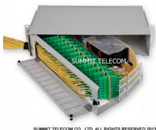
Фиг. 4. ODF(Optical Distribution Frame) 2U
